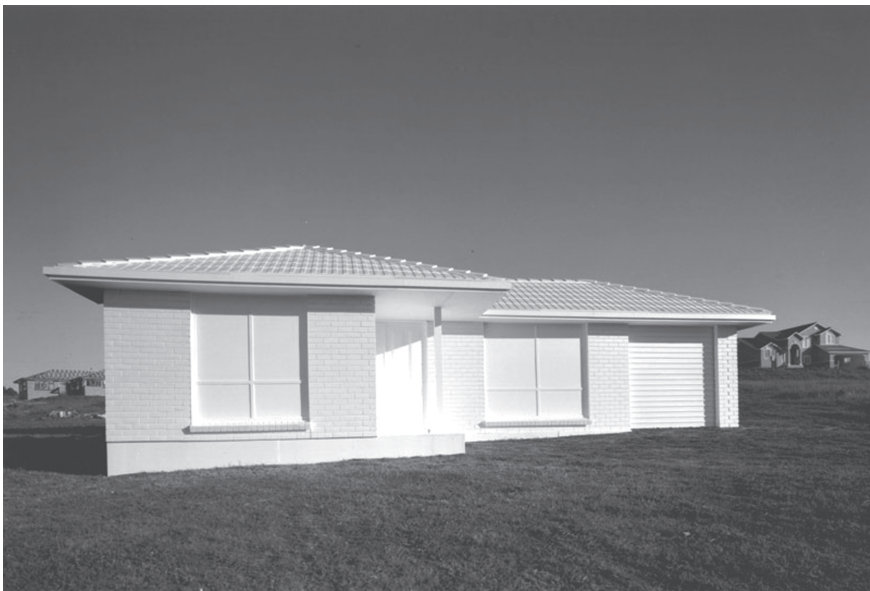
IMAGE: Mathieu Gallois Frontier (Polystyrene House) , 1998. Campbelltown neighbourhood development, Blair Athol, NSW Australia. Polystyrene. Scale 1 : 1
